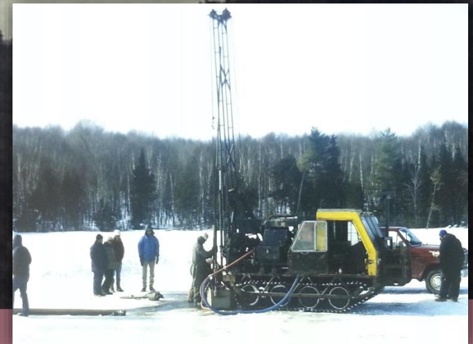
Piezometer installation through ice
